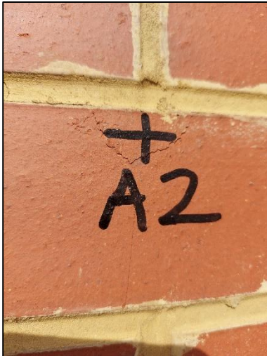
Photograph No. 9 – Damage caused following impact at location A2 Red Zone
