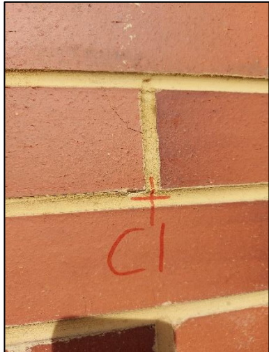
Photograph No. 5 – Damage caused following impact at location C1 Blue Zone
