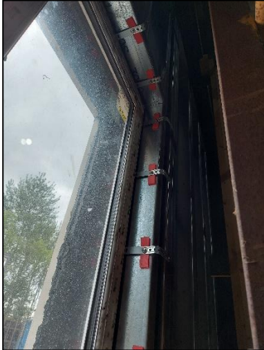
Photograph No. 13 - Internal window pod detail
