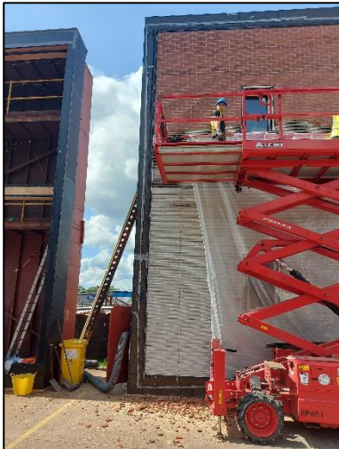
Photograph No. 17 - Sample with bricks partially removed
