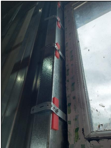
Photograph No. 14 - Internal window pod detail
