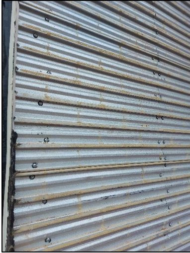
Photograph No. 19 – Backing wall and vertical rails
